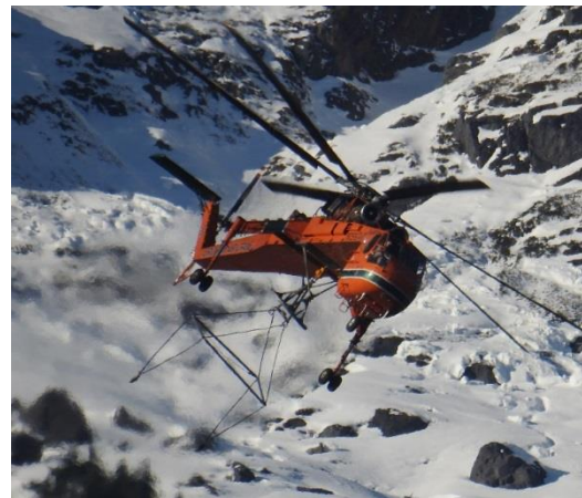
Transport of Transmission Line Structure Components
