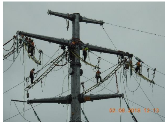
Dressing of a Transmission Line Structure
