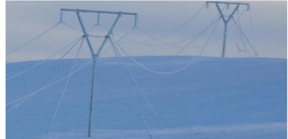
Icing on transmission lines
