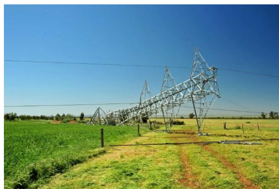
Progressive failure of Transmission lines occurred in South Australia during Sept 2016 Thunderstorms.
